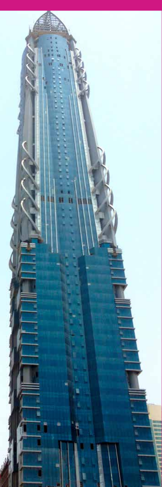
Al Hikma tower, solopix project ( Dubai ).
